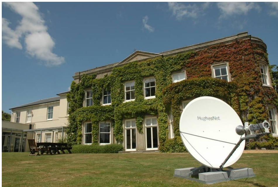
Figure 23 -The installed satellite dish outside Roke’s “Manor House” building where the user trials took place
